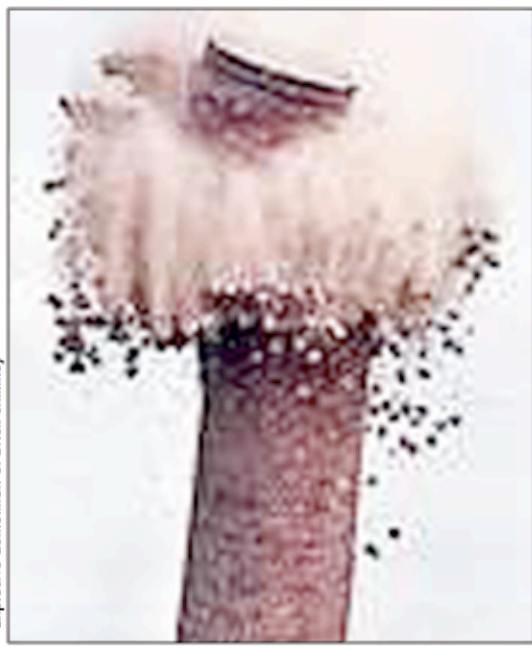
Explosive demolition of brick chimney
