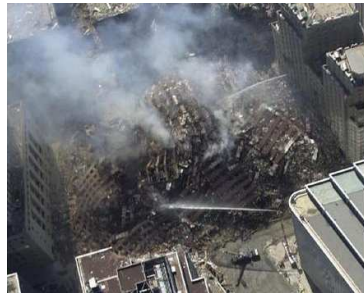
Building 7's precise fall left a tidy pile of rubble. Damage to adjacent buildings was limited, the skyscraper having miraculously avoided damaging its closest neighbors, the Verizon building and U.S. Post Office building.
