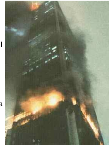
The Interstate Bank Building fire consumed several floors but did not damage the steel superstructure.
